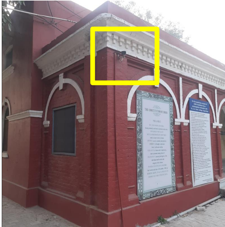
CCTV Security system in the Premises of the College.
